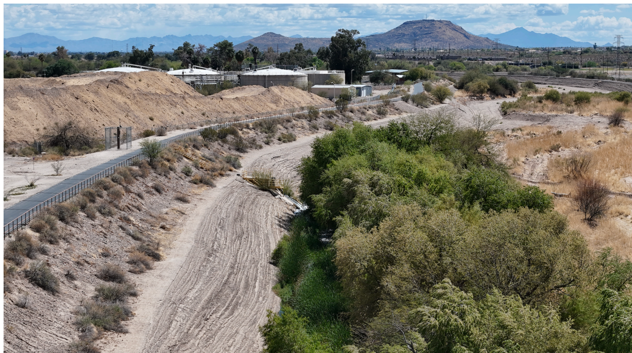
Fig. 28. Soil cement bank at Agua Nueva restricts woody riparian habitat to one side of the channel. See also cover photo for top-down view. (Photo: Rudy Malusa)
